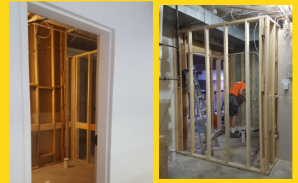
Preparations for middle floor bathrooms
