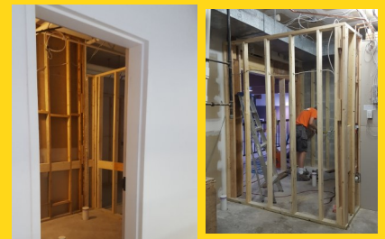
Preparations for middle floor bathrooms
